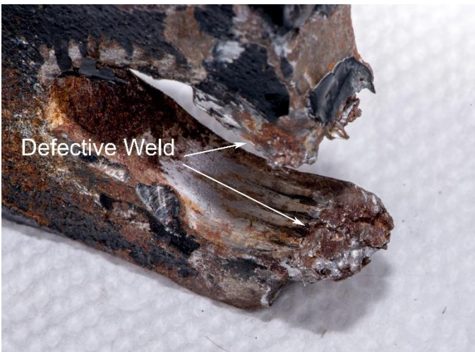
Figure 11 – Weld Porosity and Cracks on Bracket
