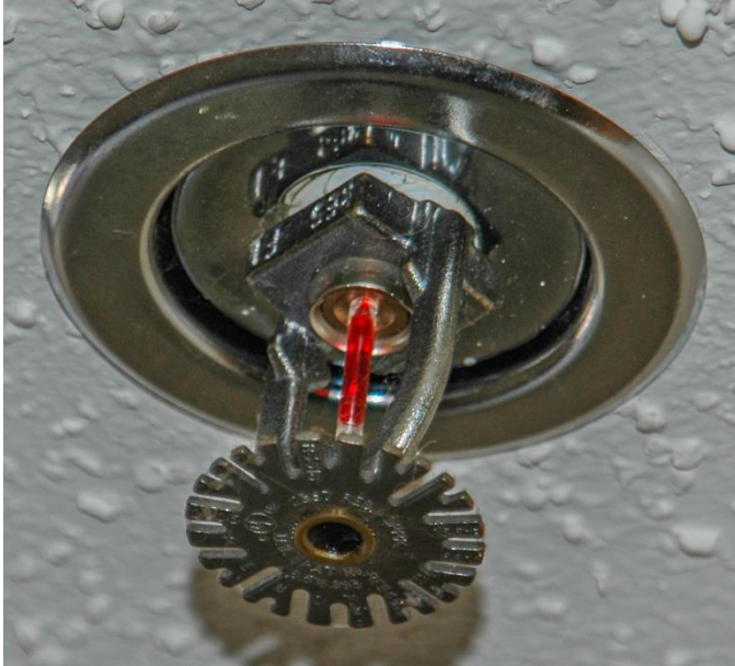
Figure 3 – Hallway Sprinkler
