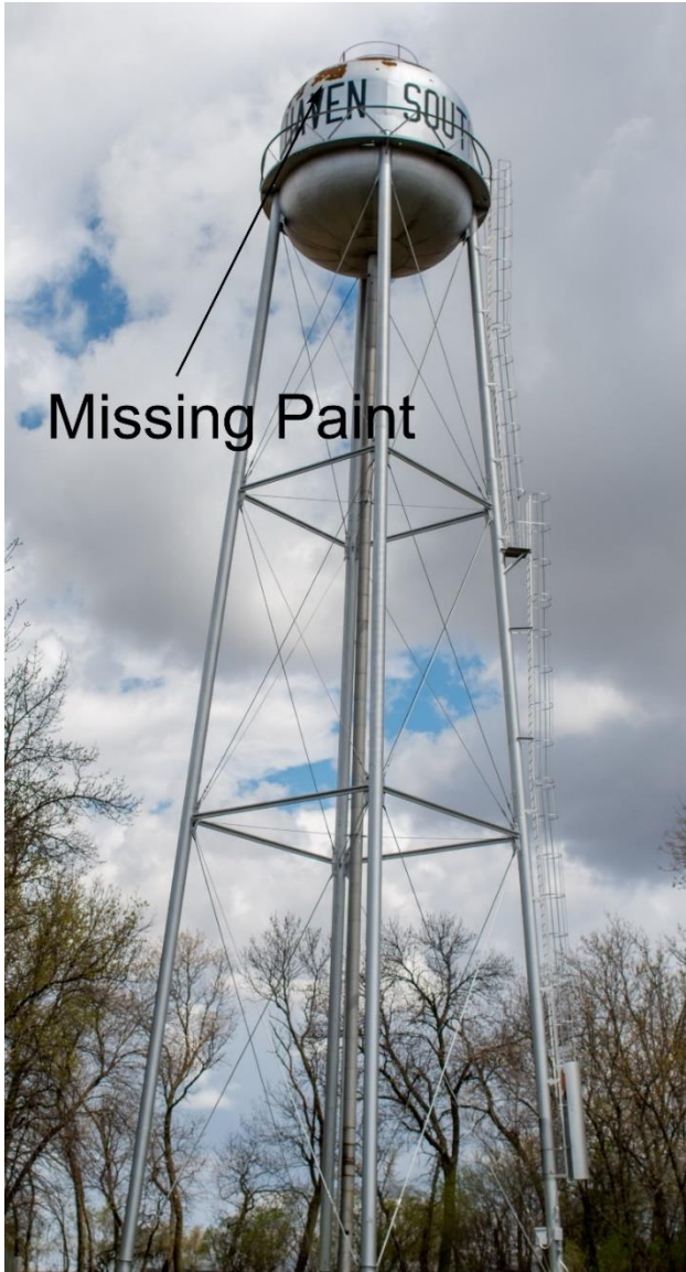
Figure 1 – Water Tower Overview
