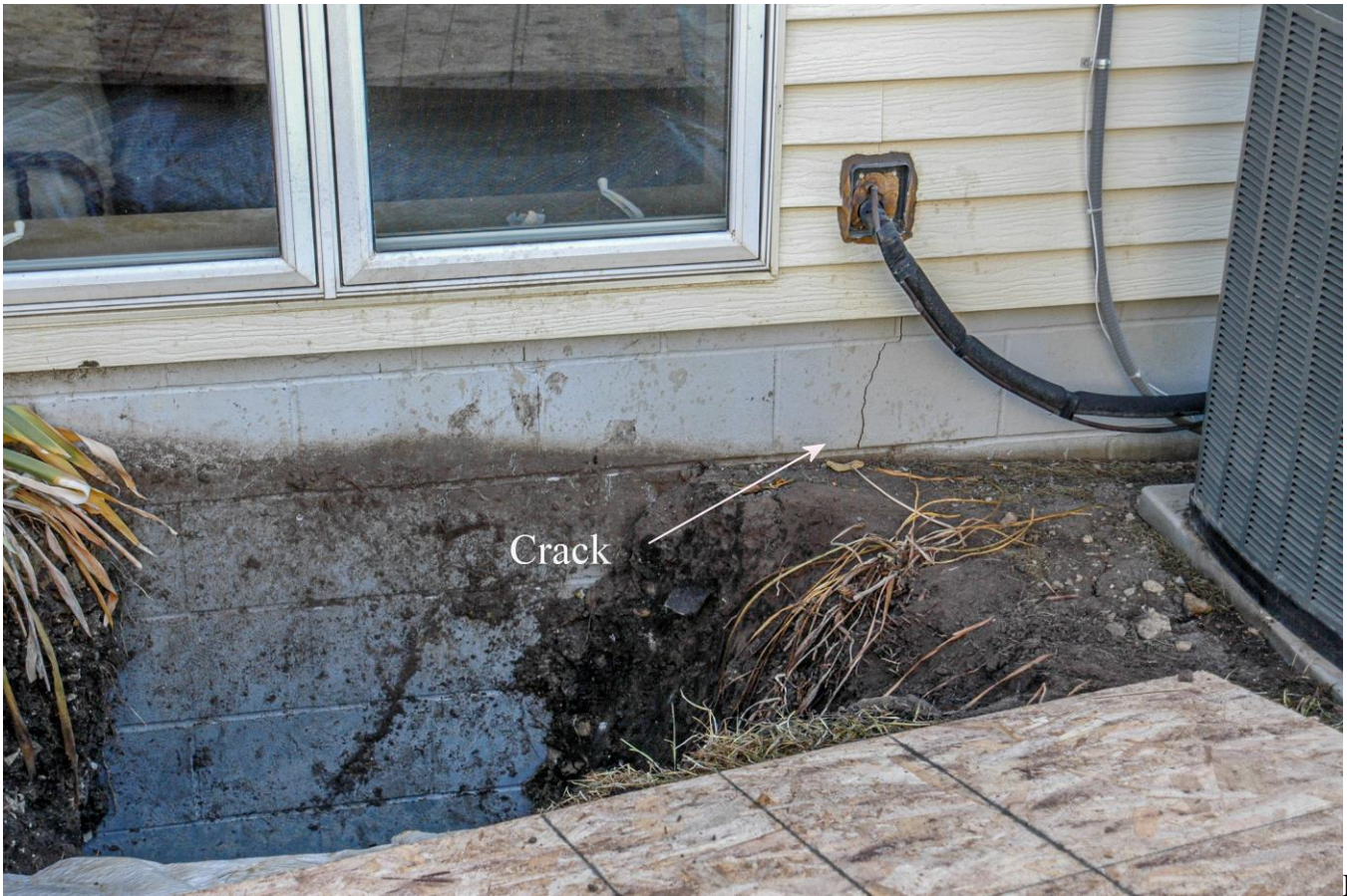
11 – Crack in Block Foundation West Side of the Home
