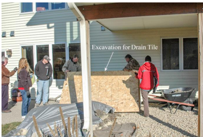
Figure 5 – Excavation Pit Location, South Side of the Home
