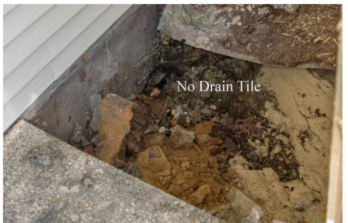
Figure 6 – Excavation Pit South Side of the Home
