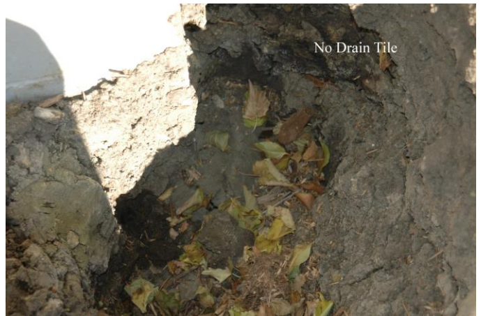
Figure 4 – Pit, Southeast Corner of the Home
