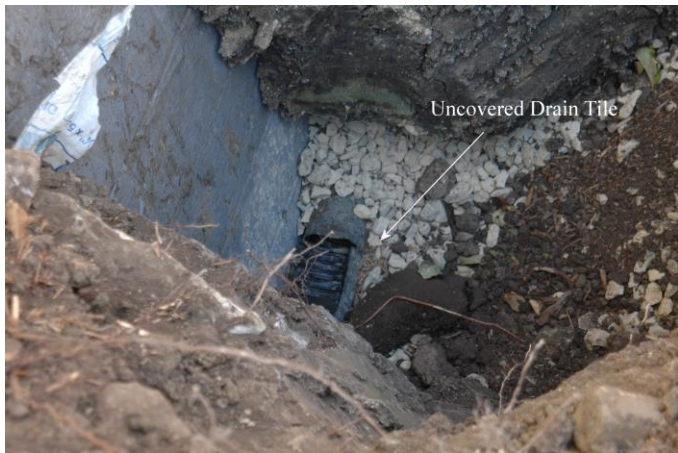
Figure 3 – Drain Tile, East Side of the Home
