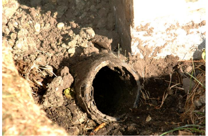
Figure 8 – End of Drain Tile Southwest Corner of the Home
