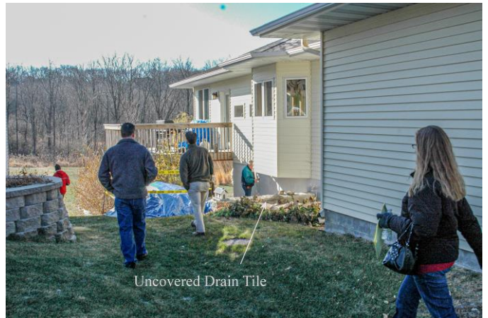
Figure 2 – East Side of the Home
