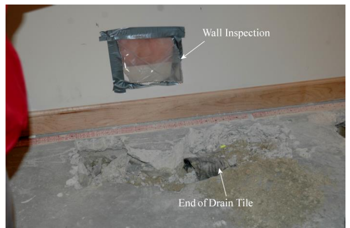
Figure 13 – West Drain Tile along Inner West Wall in Northwest Bedroom
