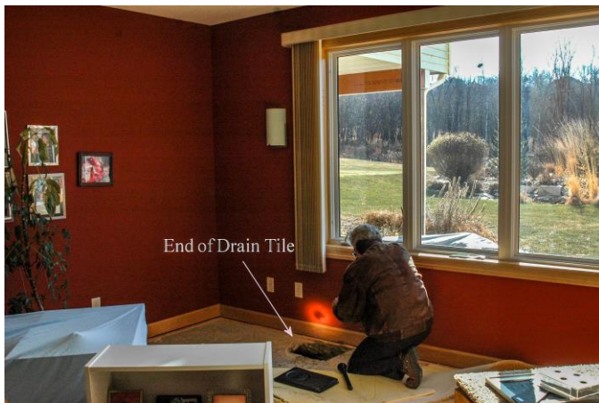
Figure 14 – East Drain Tile, South Wall
