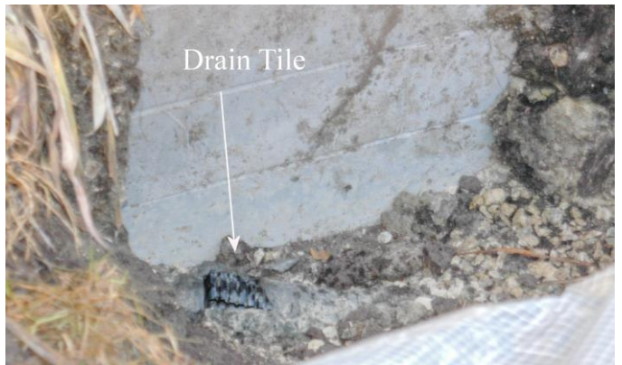
Figure 10 – Drain Tile West Side of the Home
