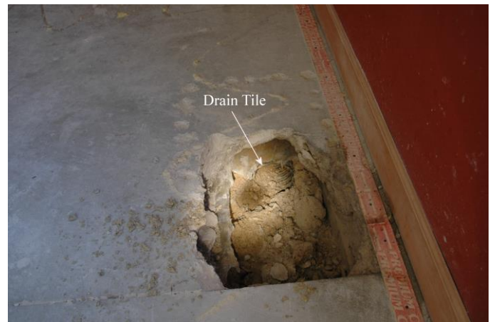
Figure 15 – End of East Drain Tile, South Wall
