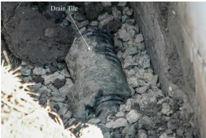
Figure 9 – Drain Tile West Side of the Home
