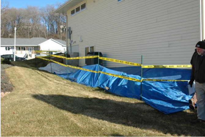
Figure 7 – Excavated Area West Side of the Home
