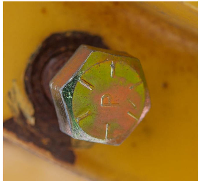
Figure 9 – Grade 8 Bolt Head
