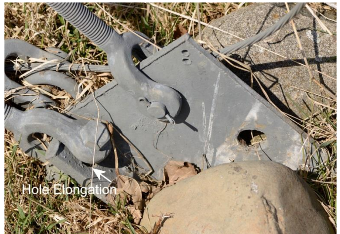
Figure 10 – East Guy Wire Anchor #2
