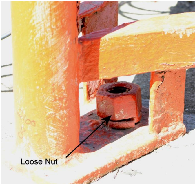
Figure 3 – Anchor Point, South Tower Leg
