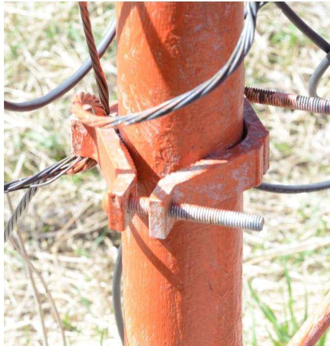
Figure 11 – Tower Ground Connection
