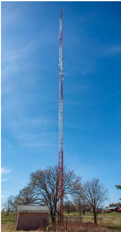
Figure 1 – Tower and Communications House
