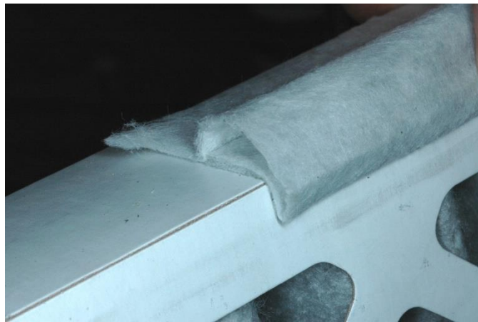
Figure 3 – Effective Seal – made from Filter Media
